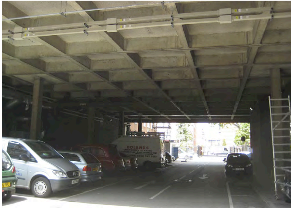
Ground floor, view from Kell Street (before)
