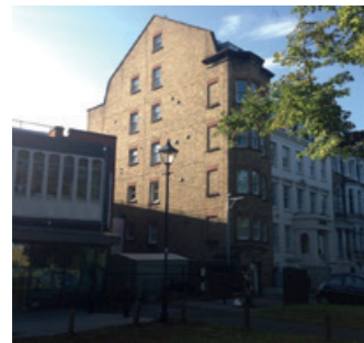
Directly adjacent to the site the terrace is terminated on a 20th century construction of seven storeys. This comprises five full floors and a double mansard of two storeys. Windows on the gable elevation will need to be considered; one line of windows appears to serve a staircase but the second line of windows may serve habitable rooms. Rights of light, daylight and sunlight will need to be assessed in terms of the impact of new development on these windows.
