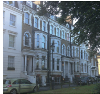
To the south of the site on the A24 are grand five-storey nineteenth century terraced dwellings. These define the building line and are the dominant historic scale in the area. These have three full floors plus a lower ground and one or two mansard storeys. Service road and green verge provides a good foreground view and welcome separation from traffic.
