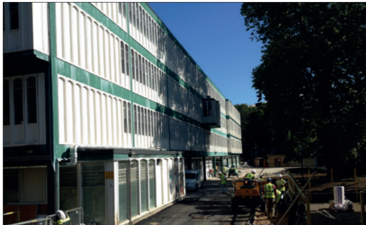
Block C viewed from the south
