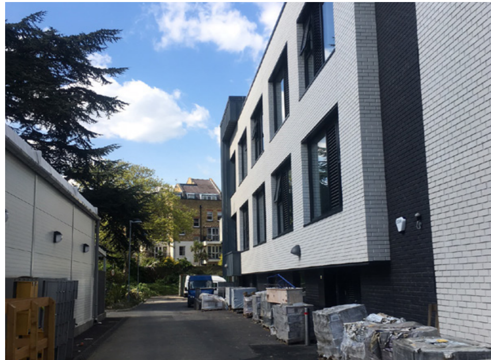
Rear of Henry Thornton Building
