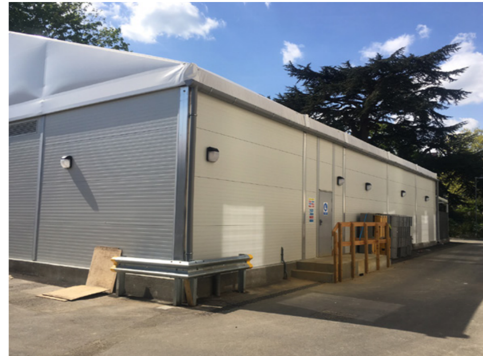
New Temporary Construction Accommodation
