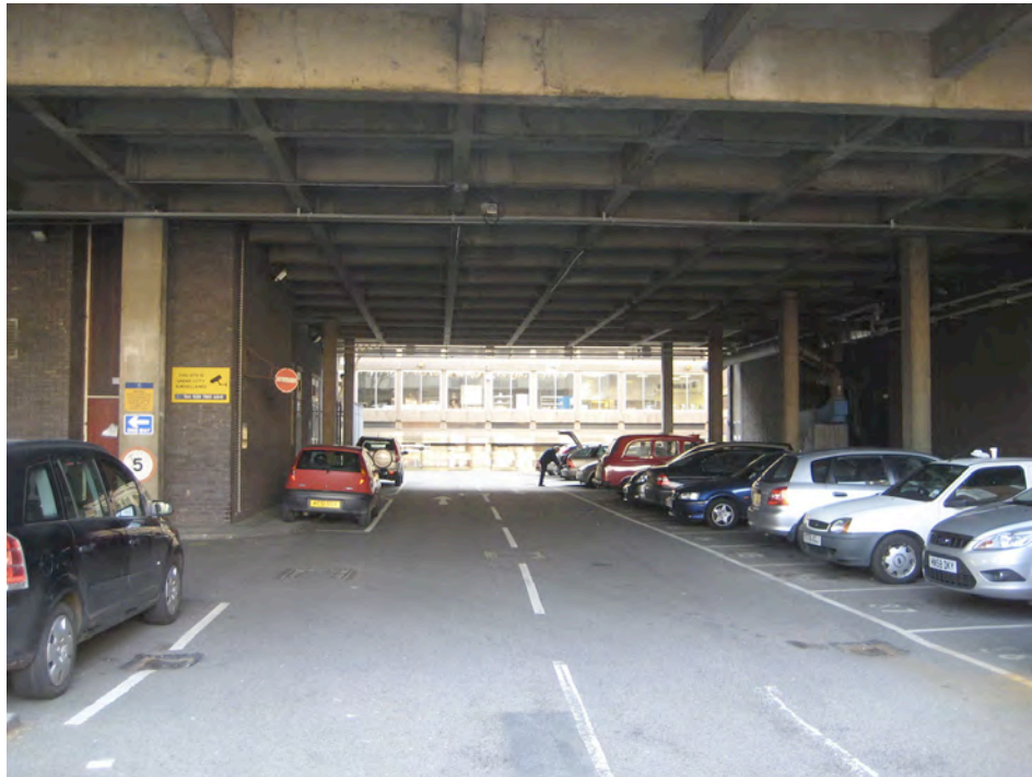
Ground floor, view from Borough Road (before)
